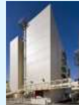
NIPPN's Kobe-Konan Mill Completion of grain silo in Jun. 2012 Completion of a flour milling line in Sep. 2012
